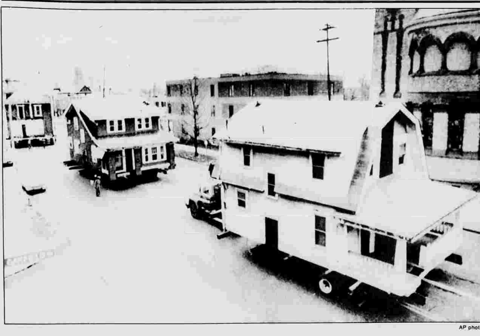
MOVING EXPERIENCE — A parade of houses on wheels moves along Broad Street in Columbus, Ohio, Saturday. They're the first of 20 houses that are being moved to city-owned lots for renovation and sale to first-time home buyers.
